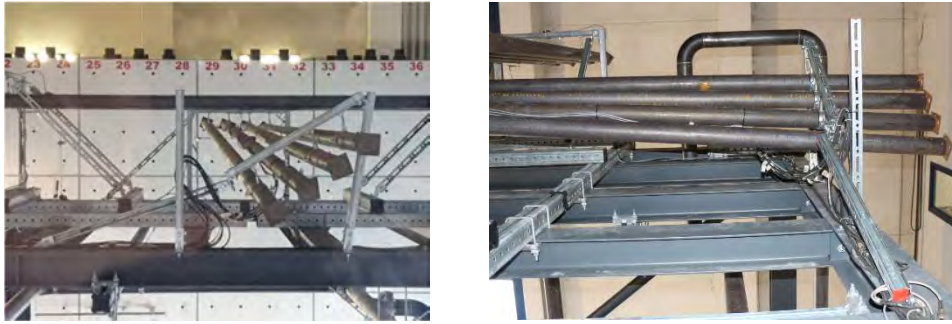
Figure 92: Damage of suspended pipes at 3rd floor
