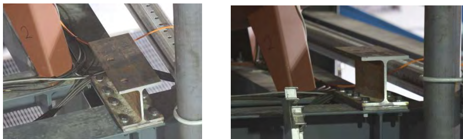
Figure 94: Strengthening: Additional profile connected to the cross and frame beam by bolts - Tank 2
