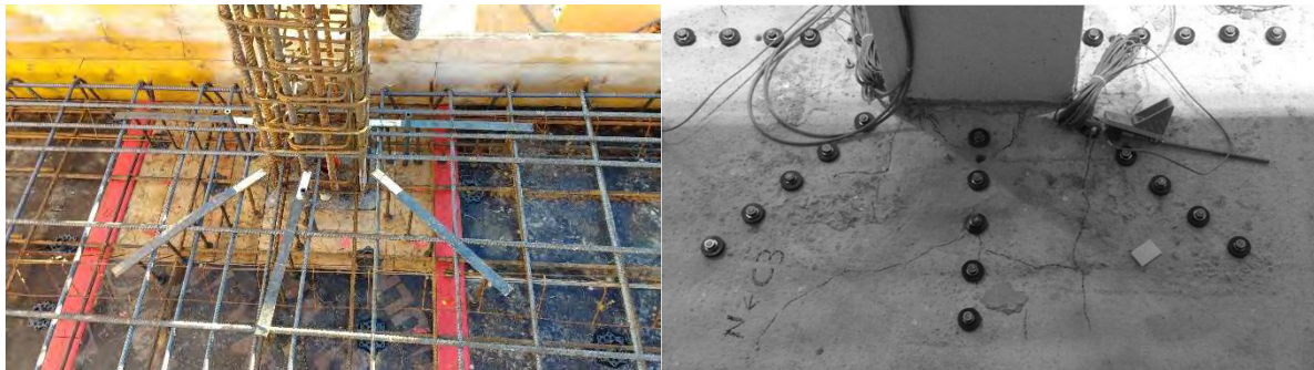
Figure 22: Shear reinforcement on edge columns: pre-installed at second floor (left) and post-installed at first floor (right)
