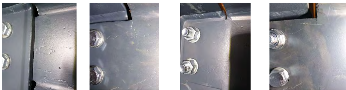
Figure 95: Cracks in the web of the cross-beam (100%)
