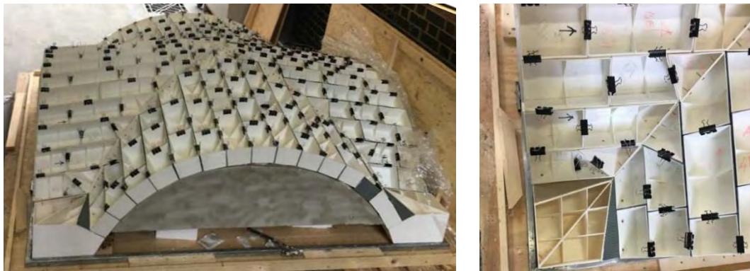
Figure 306: Pre-assembly of the plastic skin of the blocks
