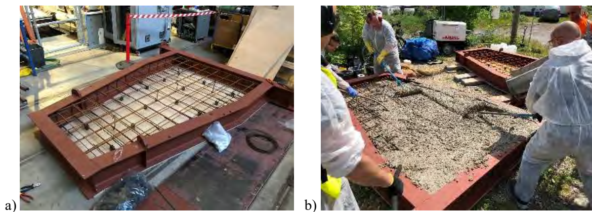
Figure 271: Working phases of base construction: a) addition of rebar mesh and b) concrete casting
