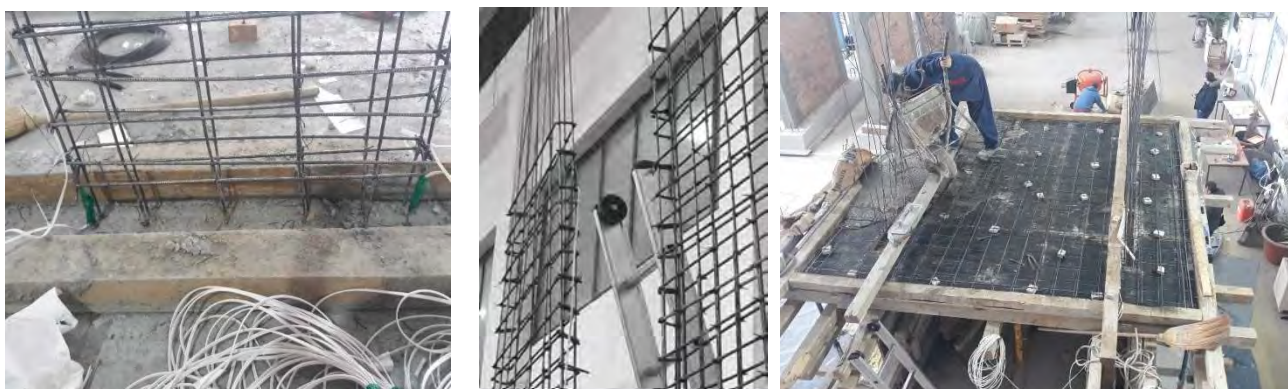
Figure 346: Mounted reinforcement in the bearing walls (left) and slab concreting (right)
