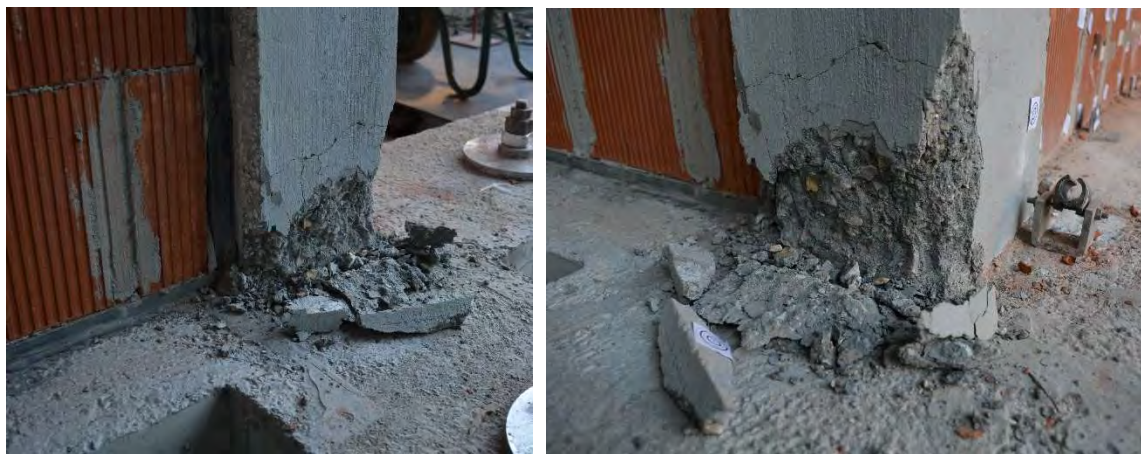
Figure 405: Spalled concrete cover of the column in the bottom
