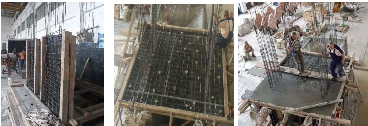
Figure 361: Mounted reinforcement in the bearing walls (left) and slab concreting (right)
