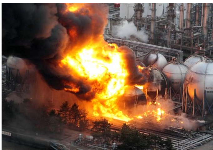
Oil refinery in Ichihara after Fukushima earthquake
