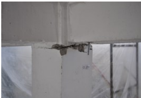
Cracking at column-foundation and column-joint interfaces of the first floor
