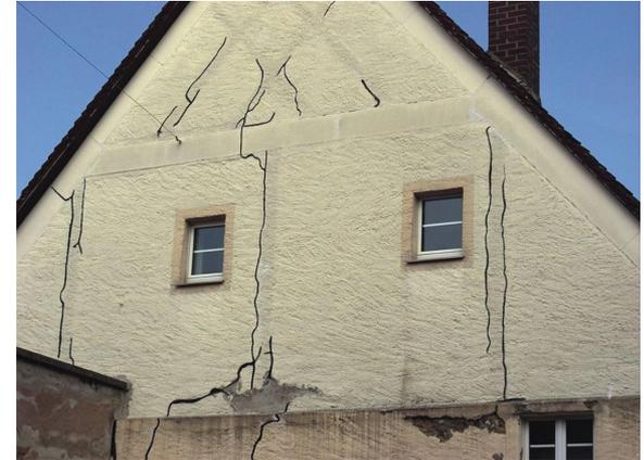
Fractures in building wall after the 3.4 mag. eq. in 2006 beneath Basel (source:www.bazonline.ch)
